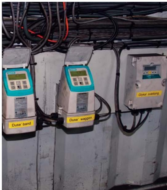
SITRANS F M MAG 5000 (left and middle) and SITRANS FST020 flowmeters (right) accurately measure and control glycol and water used to prevent coal from freezing.
