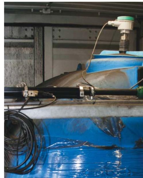
SITRANS FST020 clamp-on flowmeter sensor (left) controls glycol, while SITRANS LC300 transmitter (right) monitors its level in the storage vessel.
