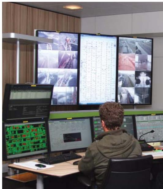
Using SIMATIC S7 control system, operators monitor everything – from ship traffic to machinery to instrumentation – from the comfort of the control room.
