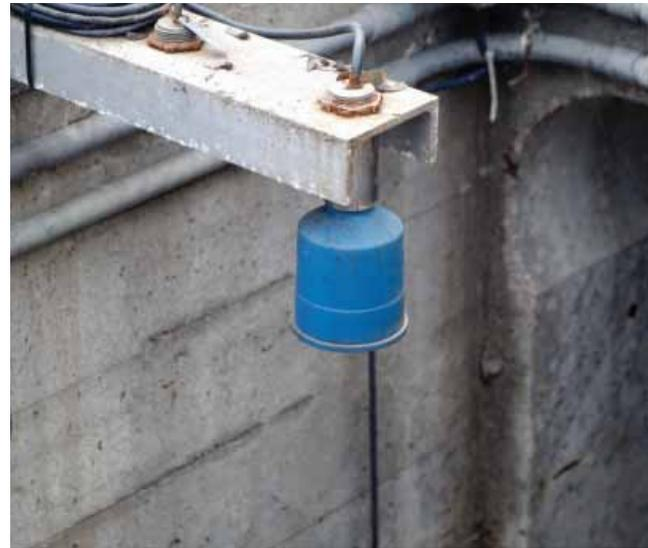
With millions of liters of water treated, this municipal water system relies on the accuracy and reliability of SITRANS LUT400. The SITRANS LUT400 is compatible with the full range of Echomax ultrasonic transducers from Siemens.
