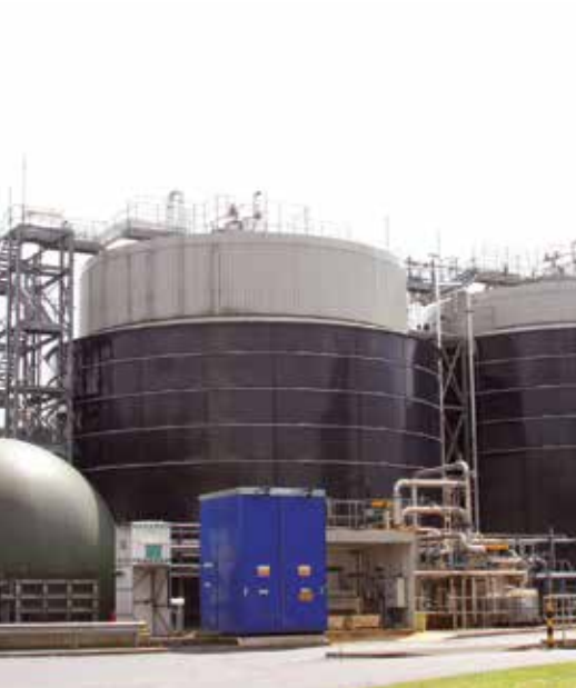
The two massive anaerobic digesters tower over the finished biogas gasholder.
