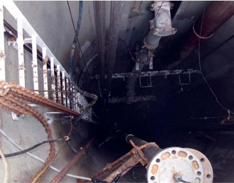
With the numerous obstructions in this wet well, including a ladder, pipes, and chains, accurate and reliable level measurement can be quite challenging.
