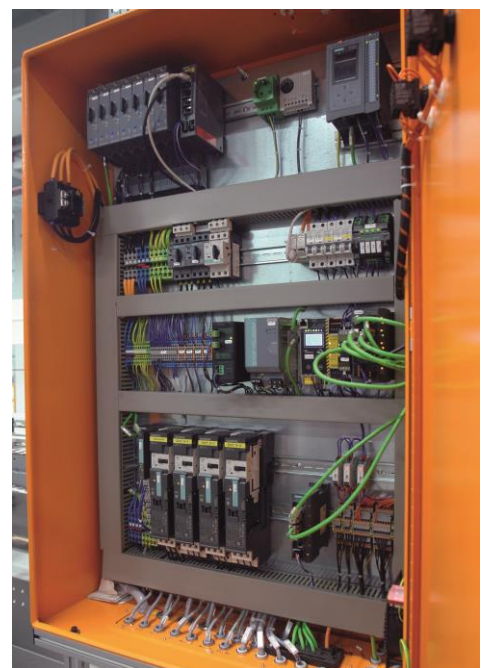
The space requirement makes all the difference: the new ET 200SP motor starters save about two thirds of the space in the control cabinet taken up by the previous ET 200S solution.
